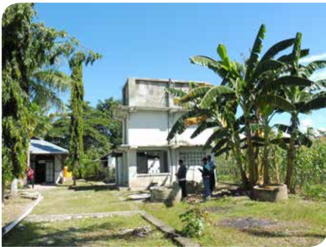
Water reservoir (on the roof).
