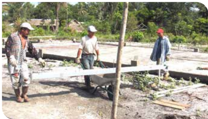
The steel structure was erected in 3 days.
