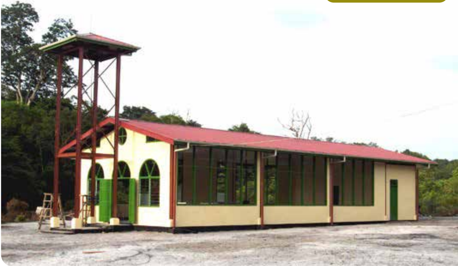
The new church.
